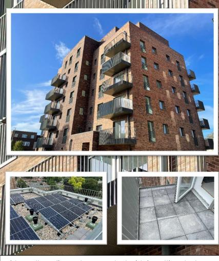
Ridgewell Roofing Ltd were tasked with installing the hot melt and liquid waterproofing and finishes to the main roofs, lift overruns, terraces, balconies and canopies on 3 nr new build blocks. Finishes consisted of insulation, pebbles, slabs on pedestals, lead work and all aluminium cappings and rainwater goods from the roofs down to the ground floor.
