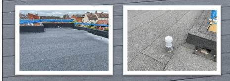
A challenging project where 2200 m<sup>2</sup> of defective roof coverings over numerous areas had to be stripped and renewed, whilst maintaining waterproofing integrity to ensure that all the shops below could remain in full operation. Once stripped, new plywood upstands and cappings were formed so that the parapet was enclosed and a new warm roof bituminous system was installed.
