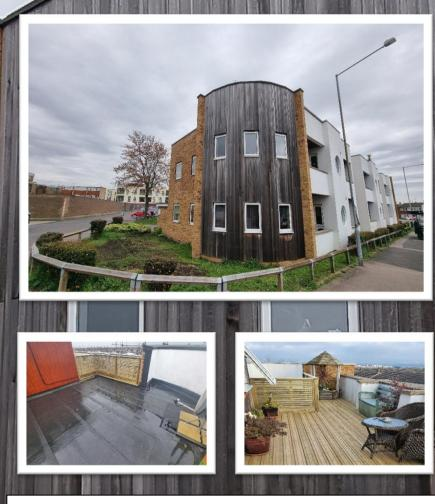
Acting as Principal Contractor Ridgewell Roofing Ltd erected scaffold and temporary roof over one section of the building to facilitate the parapet demolition, re-construction and roof replacement works. Once the waterproofing works were completed, new timber cladding, decking and fencing was installed, along with new coping stones where required, render repairs and re-decoration works.
