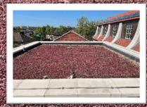
Working in partnership with Bauder, Ridgewell Roofing Ltd designed, supplied and installed new waterproofing systems to various roof levels over two phases. Works included three layer felt with insulation, cold applied liquid sedum blanket green roofing with pebble margins and slabs to private balconies. Lead work and drainage installations also formed part of our package.
