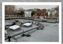
As the appointed Principal Contractor, Ridgewell Roofing Ltd provided scaffold, welfare, storage and lifting facilities. Working closely with specialist subcontractors the existing cold-water feeds were disconnected, redundant feeds removed and the remaining raised to accommodate the new roofing system and insulation thickness. New bathroom extract systems were also installed.
