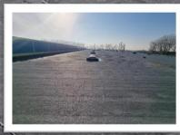
Ridgewell Roofing Ltd were appointed as Principal Contractor to install 6,500 m² of Bauder waterproofing along with 1,600 lm of Delcote gutter, lap and cut edge liquid coatings. As part of the works the existing cladding was cut and adjusted to suit the new system and ensure safe2torch practices could be adhered to, along with working around the recently installed air conditioning units.
